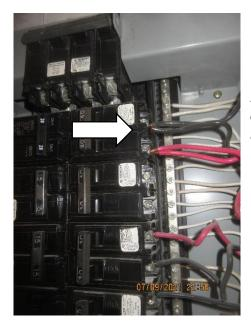
*P: the stove circuit utilizes two separate circuits that share a common 40-amp circuit breaker. An electrician should review the wiring installation for the stove.*
