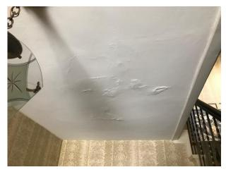
G: the water stains in the front hallway ceiling were checked with a moisture meter and found to be dry during the inspection. The damage was apparently due to an overflow from the bathroom above. 7.02 Flooring: The flooring systems show no obvious structural defects. They felt secure throughout and are functional. The staircases in the house are sound. The door jambs are relatively square, allowing good closure of interior doors. The hardware on most doors is functional.
