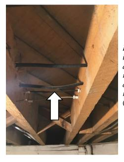
*P:* budget for replacement of all original wire. This would include the installation of additional outlets and possibly additional lighting circuits. The kitchen wiring does not require upgrade. Interconnected smoke/carbon monoxide detectors should be installed on each level as part of the rewiring.
