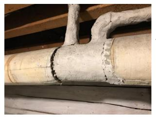
*G*: asbestos insulation is present around the rad pipes in the front basement storage room beside the basement staircase. The insulation is for the most part intact. You may however want to have it removed. The vinyl floor tiles in the basement rec room and on the basement stairs likely contain asbestos. The material is bonded within the vinyl tile and does not pose a risk if left undisturbed.
