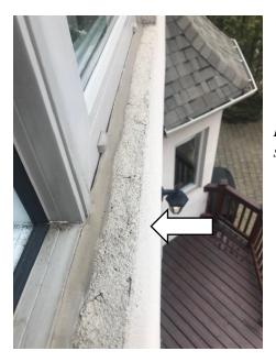
*P: the stucco has deteriorated on both rear bedroom window sills and repairs are required to ensure watertightness.*
