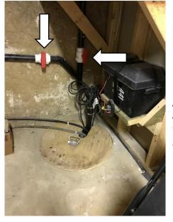
The sump pump discharges water into the waste plumbing system and also has the ability to discharge water to the exterior at the back corner of the house via a red valve that would need to be manually operated. This option should be used during warm weather conditions. 1.03 Exterior walls: The exterior walls are constructed of solid masonry. The masonry is a structural component and supports some of the load of the house. The rear addition walls are wood frame construction.
