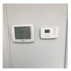
The thermostat at the west end of the  $2^{nd}$  floor hallway area controls A/C only. The humidistat beside the A/C thermostat controls the steam humidifier located in the basement.
