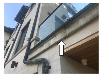
*P: there is residue on the perimeter stone finishing below some of the deck surfaces. A drip edge should be provided on the underside of the concrete deck leading edges to shed water away. This may be accomplished with the installation of a bead of caulk or preferably a recessed metal edging.*
