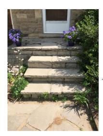
P: some of the flagstones have loosened or are uneven and should be reset on the front concrete deck structure. The missing mortar between stones should be replaced. There has been some minor movement in the deck slab and steps. Monitor.
