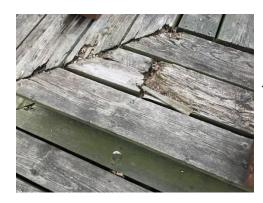
P: the NE step corner of the step structure is rotted and replacement of deteriorated boards is required. Some of the framing below the deck boards in this location may also be rotted.
